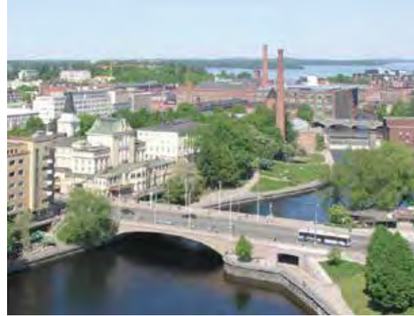
Tampere, waterlink between north- and south lakes is where Tampere grew from
