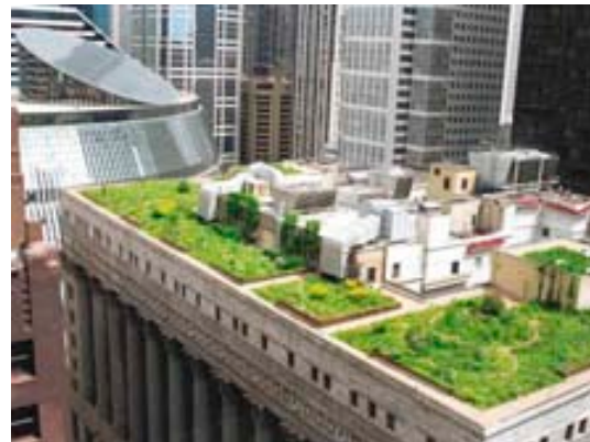
Chicago Green Roof
